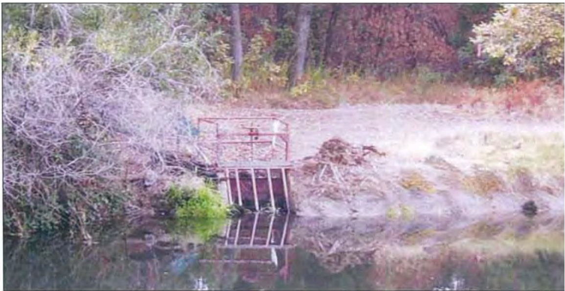
13 Diversion culvert from Auburn Ravine into Hemphill Canal
